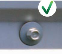
Fixed using screw PROTECT 1000™ coated with bonded stainless steel EPDM washer
