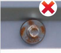
Fixed using galvanized screw with bonded galvanized washer
