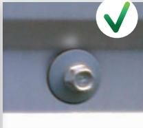
Fixed using screw PROTECT 1000™ coated with bonded stainless steel EPDM washer
